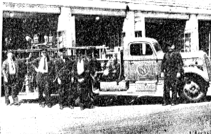
The latest addition to the Salem fire department's mobile equipment is a 500-gallon capacity booster pumper, pictured above, which all members of the department helped to build from an army truck. Standing alongside the truck are, from left to right, Capt. Ted Yarwood, Chief Vincent L. Malloy, Henry Jones, Clarence Wright and Michael Welch. Firemen on the other shift who were equally responsible for change-over task, were not present when the photo was taken.
