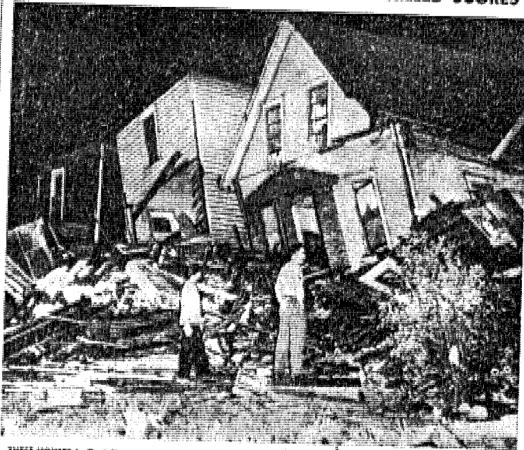
THESE HOUSES in Port Vue, Pa., were twisted and torn by the tornado that swept through West Virginia and Pennsylvania, demolishing homes, uprooting trees, and blocking highways. Eighty-six persons were said to have been killed and more than 500 injured according to early reports from the area. (International)
